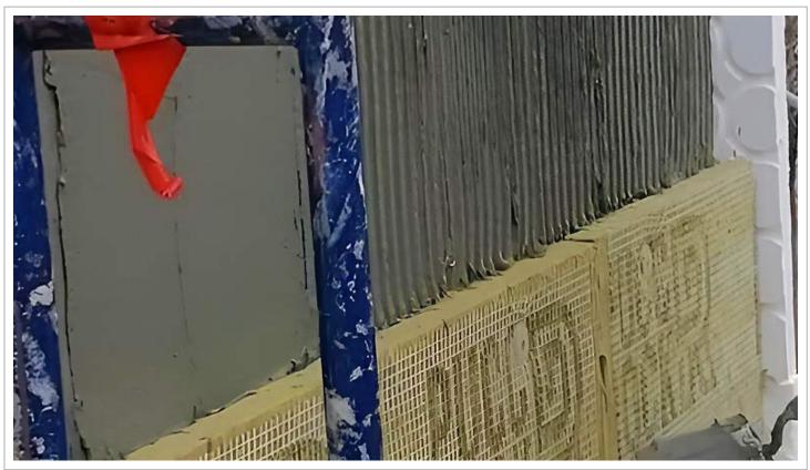
The first layer, known as the scratch coat, is applied as follows: A thick mixture of Portland cement, sand, lime, and water is prepared. The coat is applied evenly over the lath at a ¼ - ½ inch thickness. Horizontal grooves are scored into the surface for better adhesion of the next layers. The scratch coat cures for at least 48 hours under optimal weather conditions.
